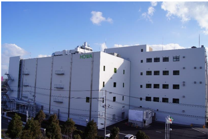
Exterior of the new factory building
